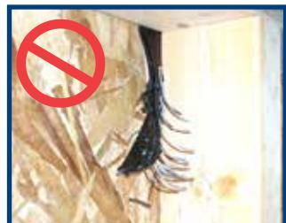
**⚠️ WARNING** Always protect hoisting straps from being cut or damaged by sharp objects such as nails, banding, cutting tools, sharp edges, hammer blows, etc.
